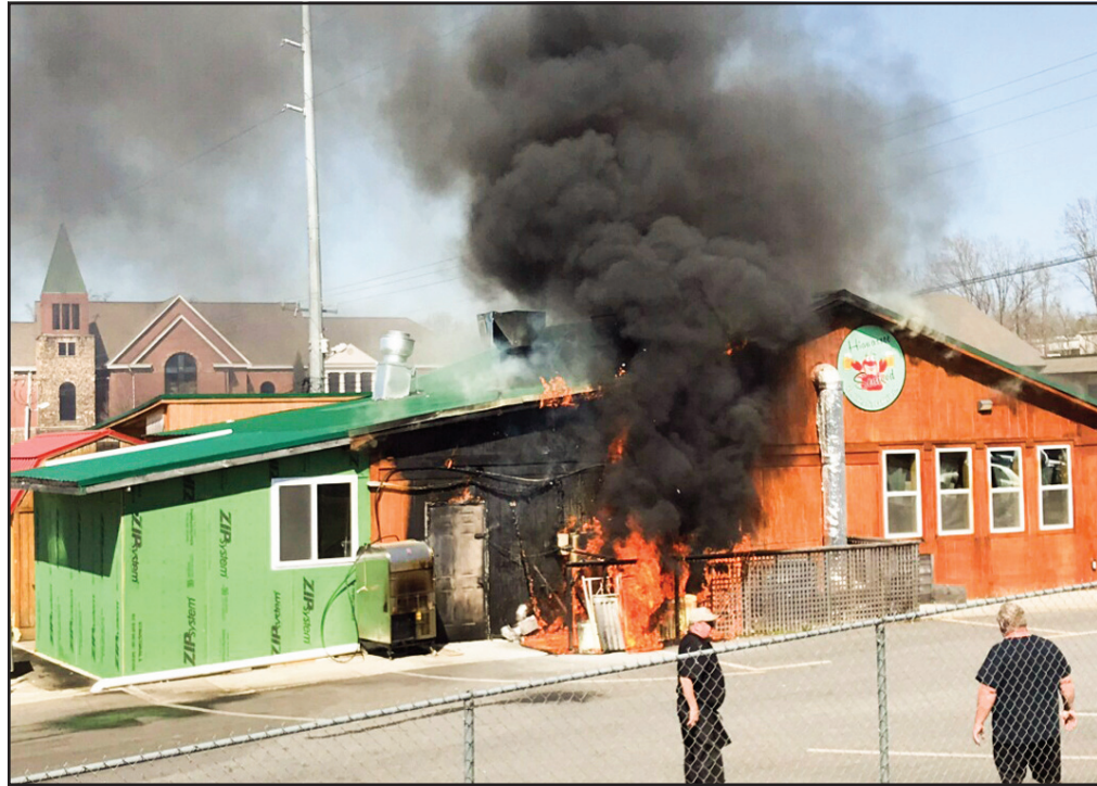
Hiawassee Seafood experienced a fire during the lunch rush Friday. Thankfully, no one was hurt, and much of the restaurant appears undamaged, though repairs are needed.
